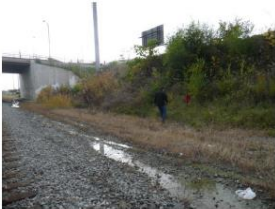
Main InterCarrier splice point north of Court Street.
