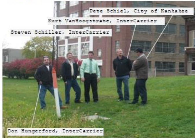
Main InterCarrier splice point south of Court Street.
